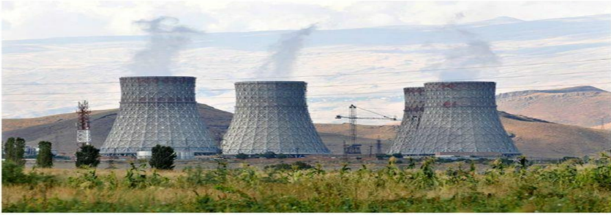
Steam rises from the cooling towers of Metsamor nuclear power station in Armenia in September 2010. One of the last old operating Soviet reactors built without containment vessels, its location in a seismic zone has drawn renewed attention since Japan's ear... Read More PHOTOGRAPH FROM AFP/GETTY IMAGES
